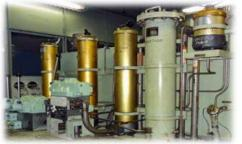
Existing mesh type filteration system could not reduce acid value
